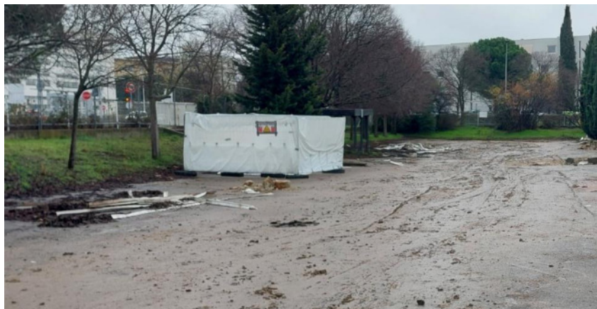
Figure 10. Example of temporary storage of asbestos waste
